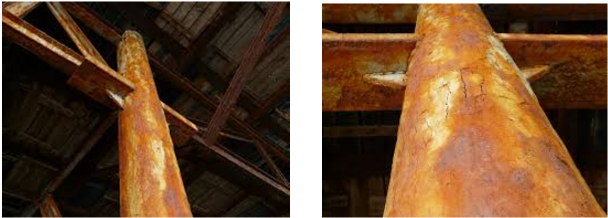
Figure 2 – Examples of corroded building structure
